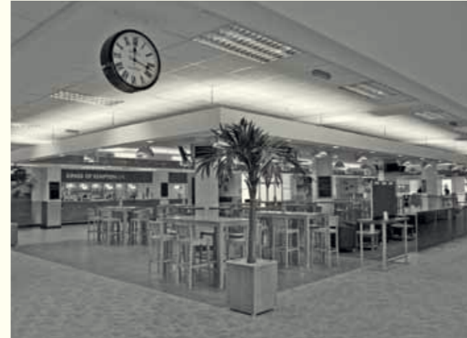
Kempton Park Racecourse Grandstand ground floor refurbishment
